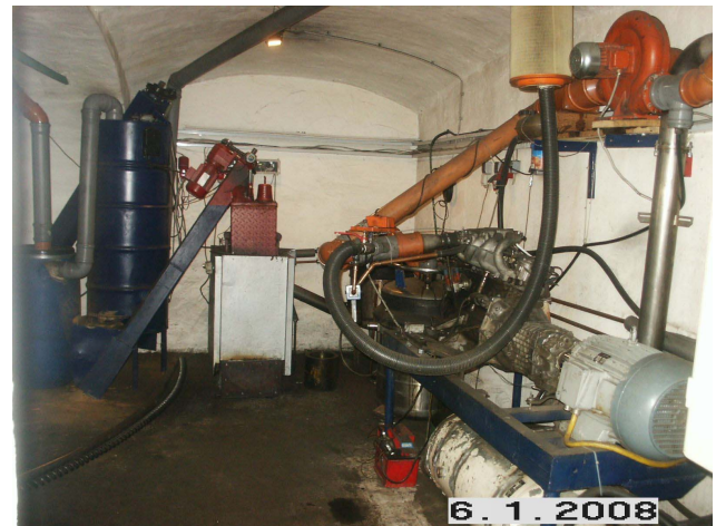
Fig. 2. The plant in January 2008.
